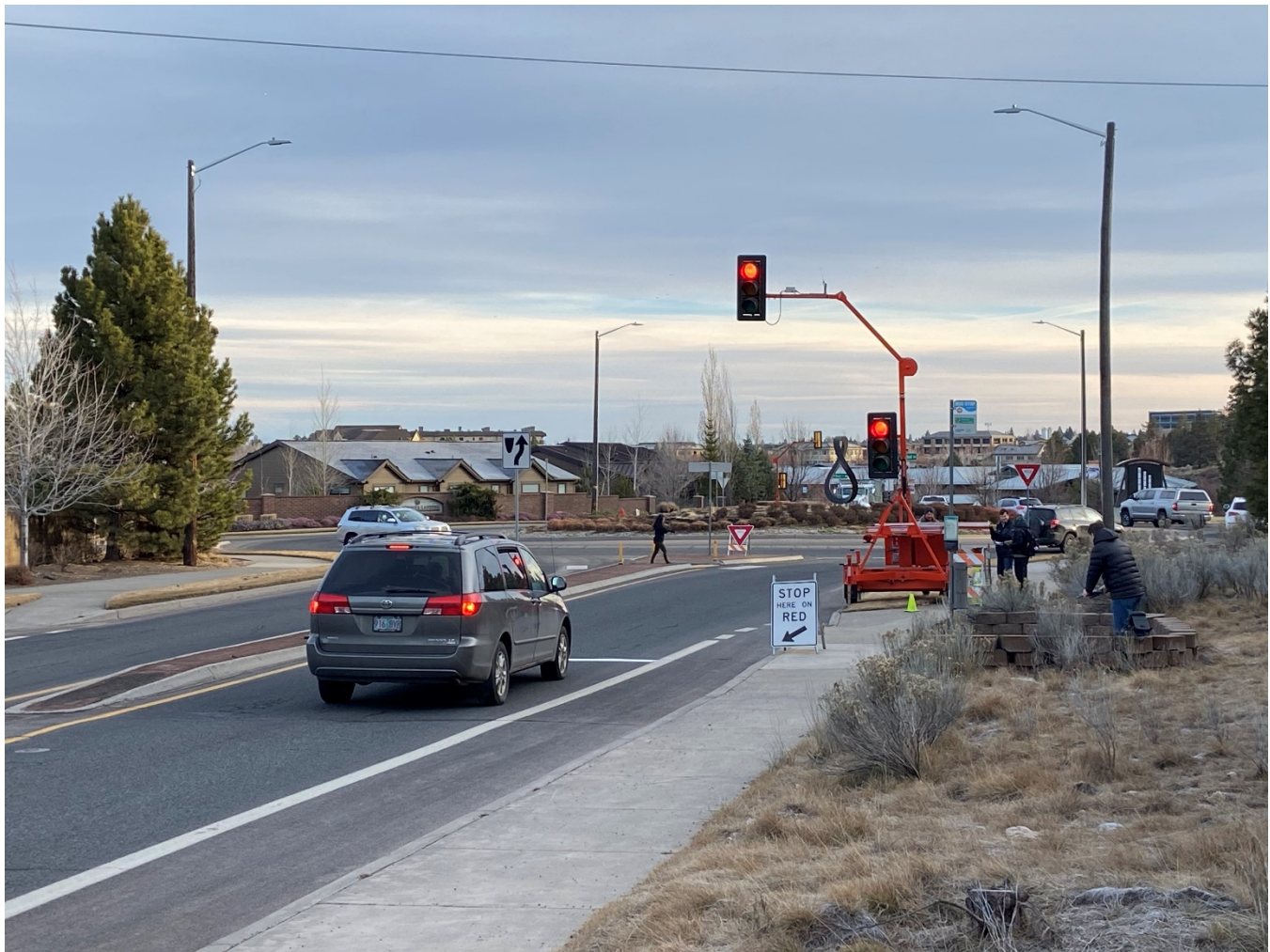
Figure 1 - Temporary Signal Set-up
