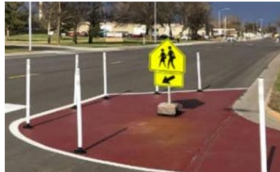
Curb Extensions – safer crossings
