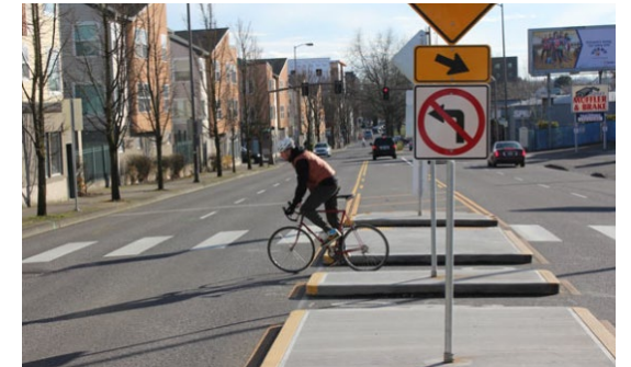
Concrete Median – Low Stress Crossing
